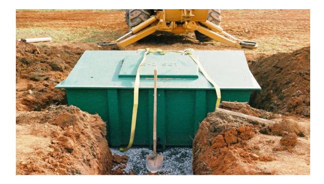
Final grading and landscaping must slope away from all tanks, riser assemblies, and the E-Z Treat Sand/Media Filter to prevent surface water accumulation.
