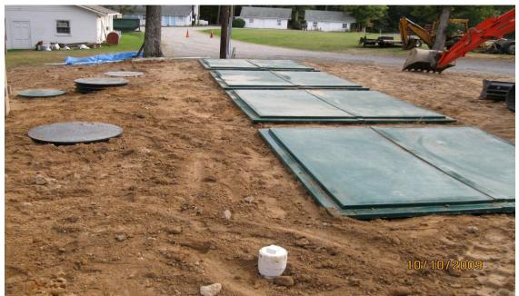
The tank opening, housing the Recirculation Pump and the Float By-Pass Valve, shall have a minimum 24-inch water tight access brought to surface level. Backfill around the Septic Tank, Recirculation Tank and Filter Pod should be done with proper care using fill material free of large rocks and debris. Remember; only backfill after tank and pipe penetrations are water tested.
